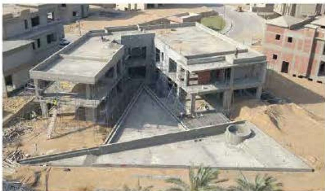
Exterior view - 60% completion of the construction phase
