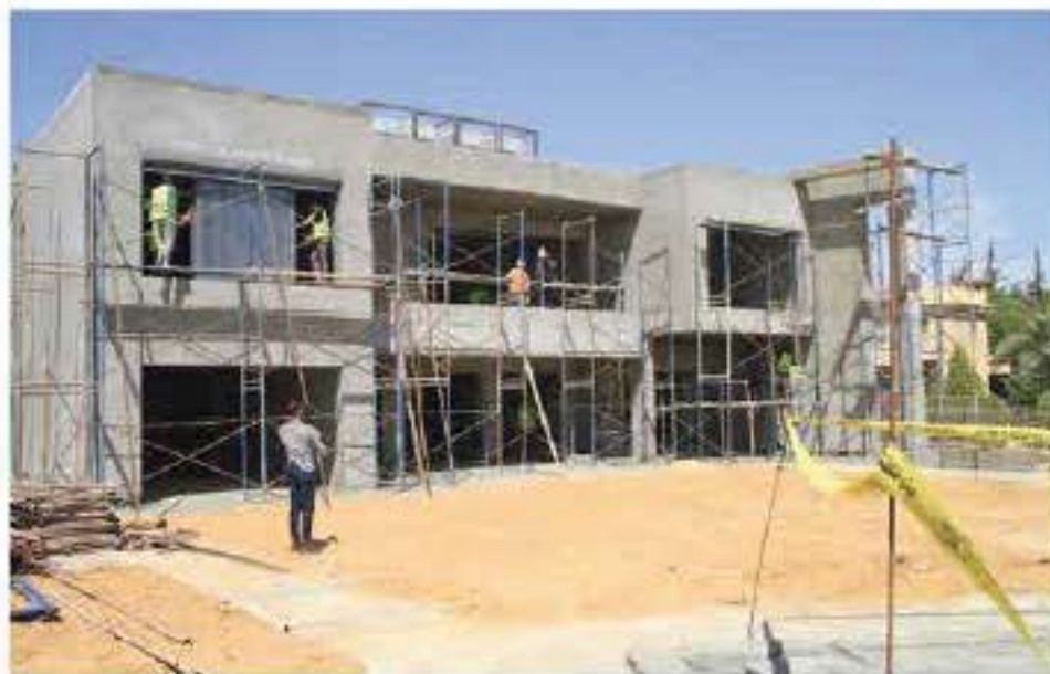
The level construction site.
