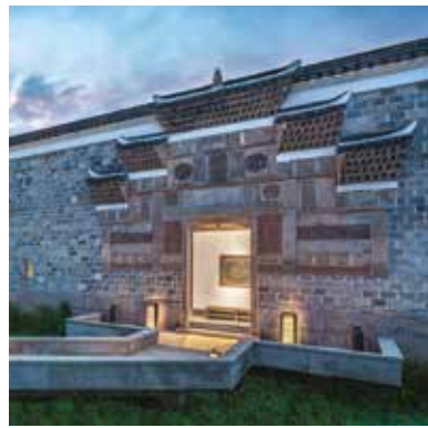
AMAN Shanghai / China Arch. Kerry Hill Architects
